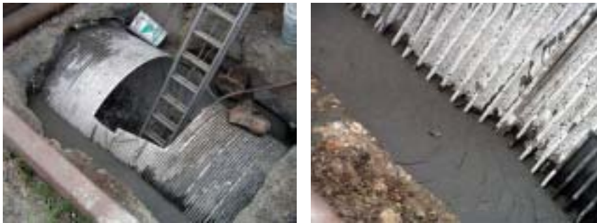
Figure 5. Partially grouted liner at 72" (1.83 m) to 78" (1.98 m) transition.
