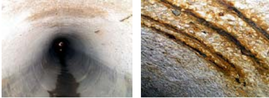
Figure 2. Host Pipe (after cleaning).
